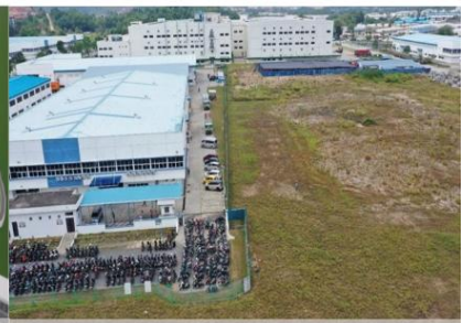
SIMATELEX PHASE 4 - BATAM
