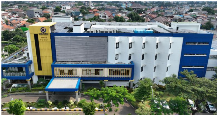
Exhibit 18. Jasamarga’s Office Building
