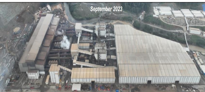
Image 19. WMI Smelter Under Construction (Sep 2023)
