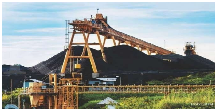
Image 15. HRUM Stockpiling & Crushing Operations
