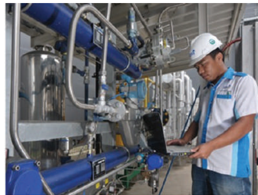
PRS Station di Customer Industry
