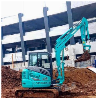
Excavator Kobelco SK50P-6 (Bucket + Breaker)
