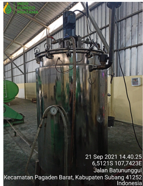
Operator Batching Plant
